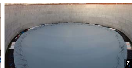
Figure 6. The detail of the tensioning system and the protective layers around the perimeter of the floating deck Figure 7. The tensioned membrane roof
